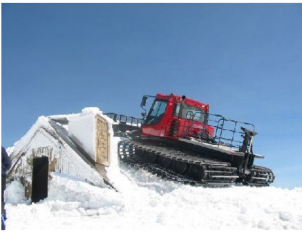
Above: Snow groomer operated by Ruapehu Alpine Lifts removing 2-3m thick accumulation of rime ice from Dome Shelter on 19 November. (Photo: Nicki Hughes)
