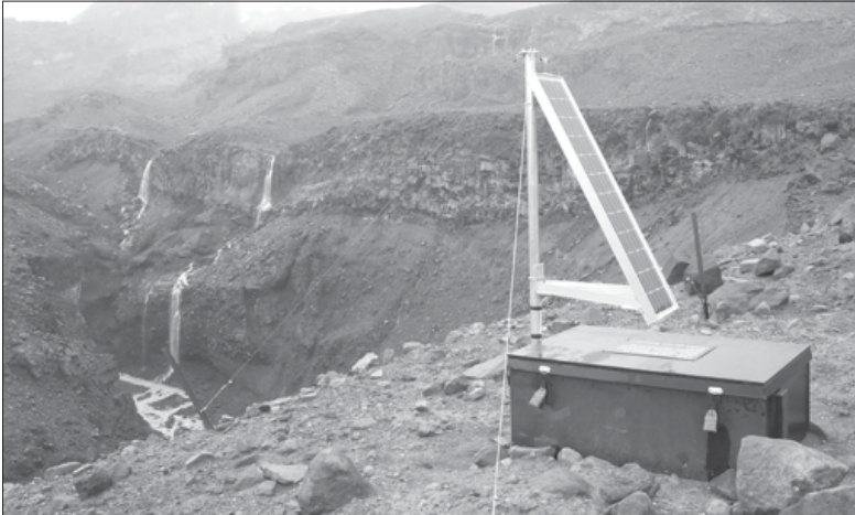
The sensor equipment at Site 3 with the Whangaehu River gorge in the background. Batteries for the equipment are charged using the solar panel. (Photo: Dave Wakelin)
