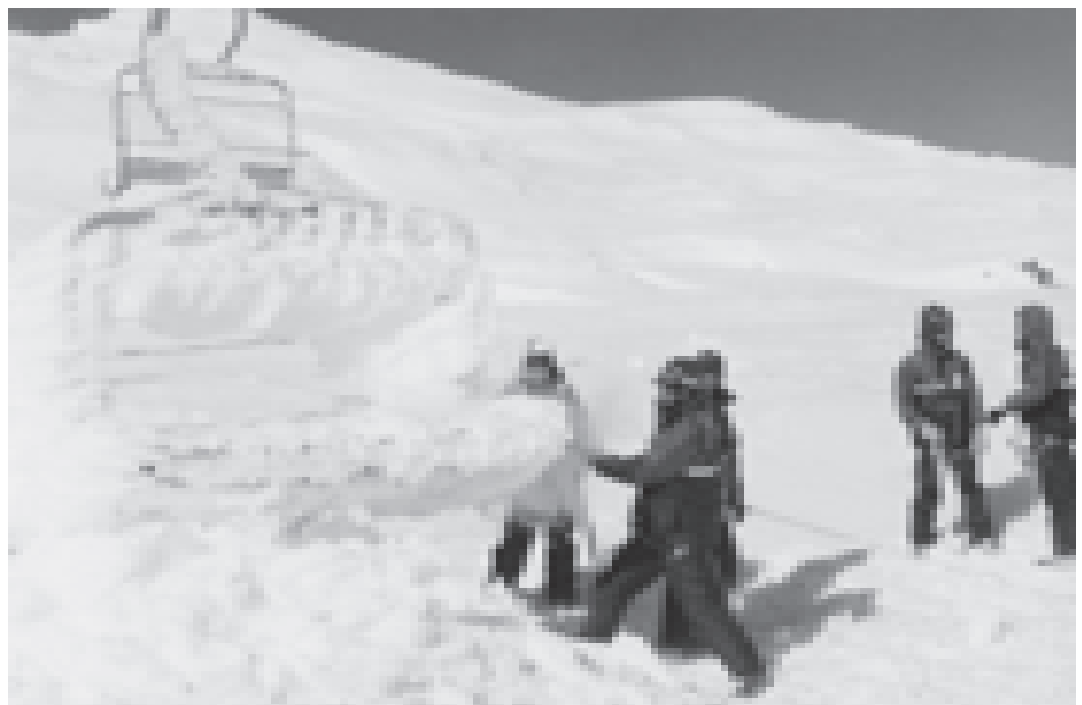
Scotty and team clearing a thick coating of rime from the West Ridge quad during the winter of 1993. (Photo: Scotty Barrie Collection)
