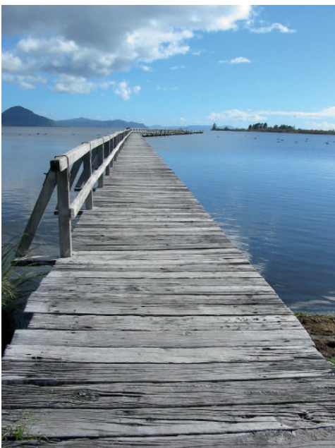
Below: The relaid first section of the wharf. Photo: Glen Hazelton
