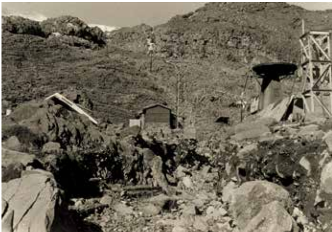
Erosion and damage to the second chair and poma at the bottom of the Staircase on Whakapapa Ski Area caused by the April 1975 lahar. Photo: Kevin Griffiths
