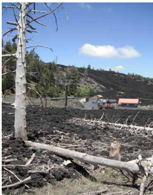
Figure 5: Lava flows in 2002 caused major damage to infrastructure and forest at Piano Provenzana (2000 m) on the northern side of Etna. There is a new chairlift and many easily moved new buildings here. Photo: Harry Keys
