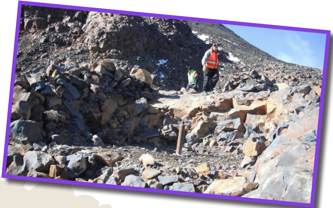
Figure 1: The completed earthworks for Matarangi as at March 2011 showing the casing exposed above the borehole. This 50m deep hole will be fitted with a downhole seismometer to detect subtle seismic data, and a tiltmeter which may allow detection of the minute inflation of the volcano that is thought to precede many eruptions. Photo: Harry Keys
