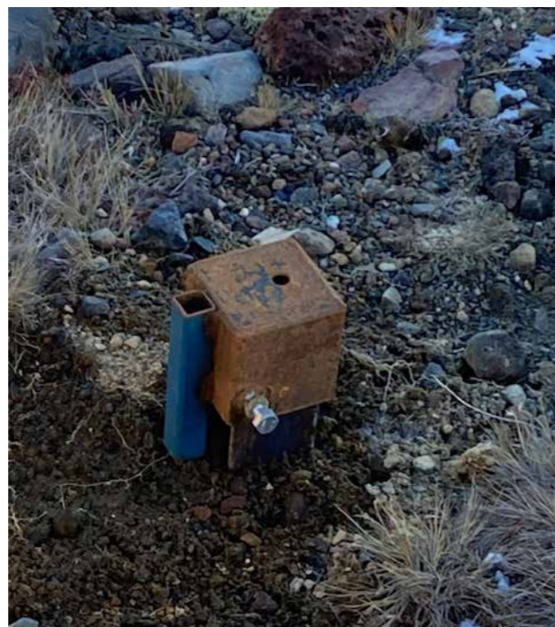
Top: A fence to keep cattle travelling up the road out of the Rongokaupo Wetland. Ruapehu Worx maintain a trapline around the wetland. Below: Boundary markers that define the Tūroa Alpine Flush surveyed boundaries. Designed by Herwi Scheltus they enable steel poles to be installed as and when needed. Left: The new Interpretation Sign at the Tūroa Alpine Flush.
