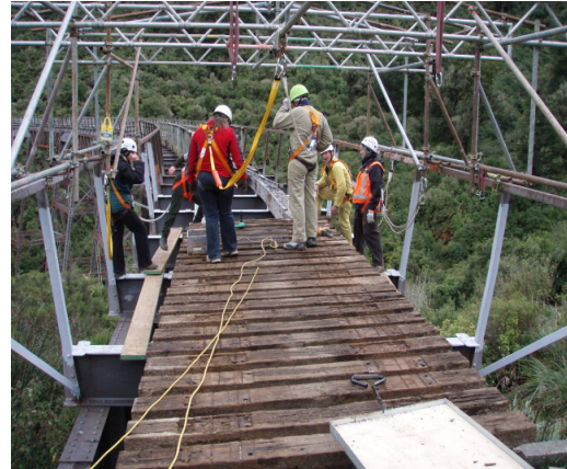
Workers are secured to scaffolding as they advance along the walkway.
